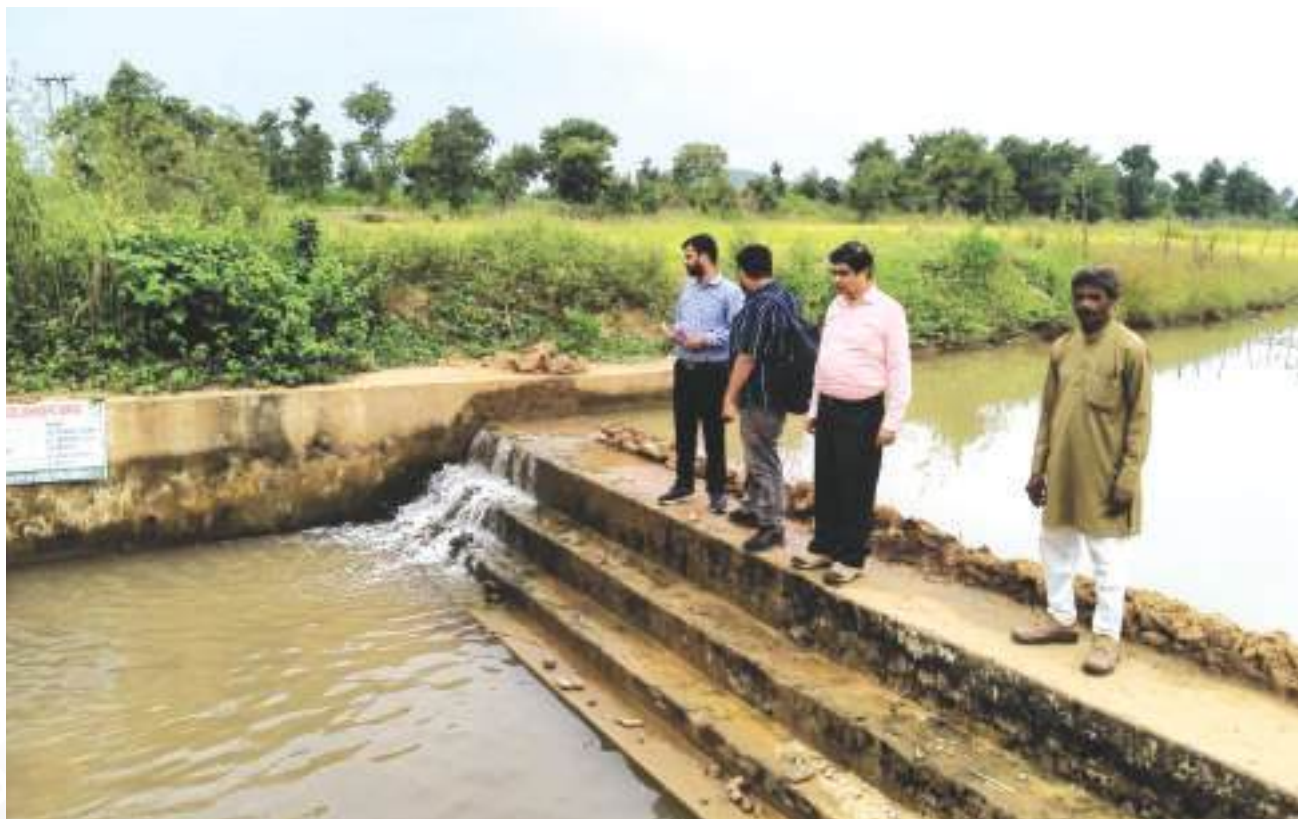
Anicut constructed under NABARD Watershed Development Project-Amriti, Distt. Satna (Madhya Pradesh)
